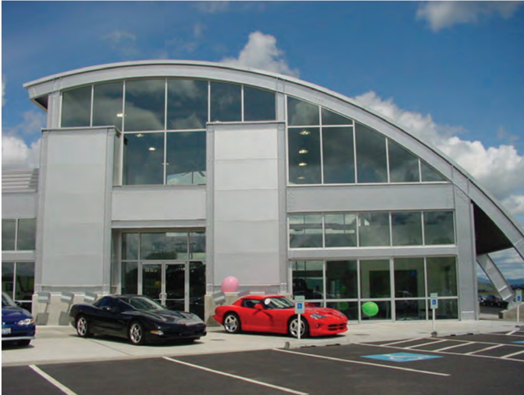
Fig. 1-2. Vertically curved roof for a car dealership (courtesy of AISC Bender/Roller Committee).
