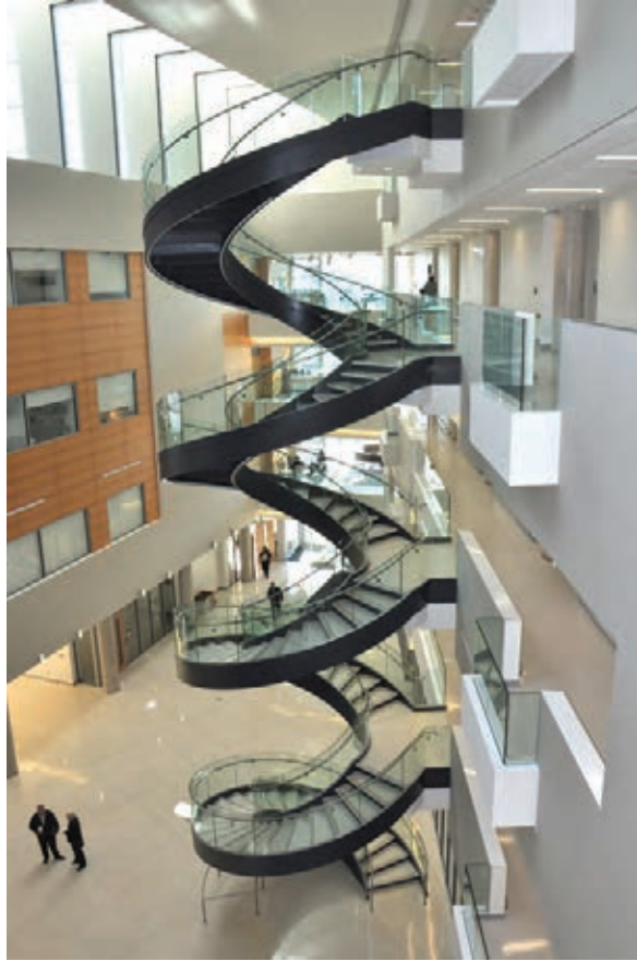
Fig. 1-10. Spiral staircase (courtesy of AISC Bender/Roller Committee).
